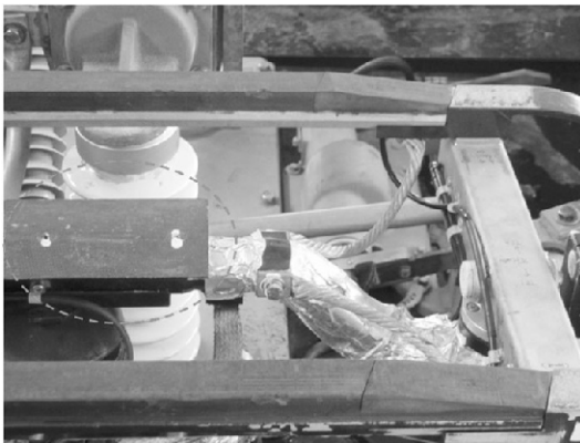
Fig. 15 Lifting control plate and contact plate
